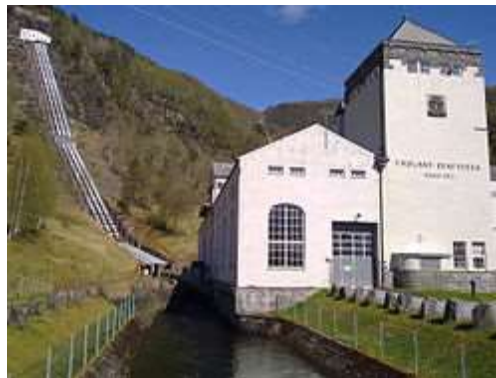
Frøland power station.
