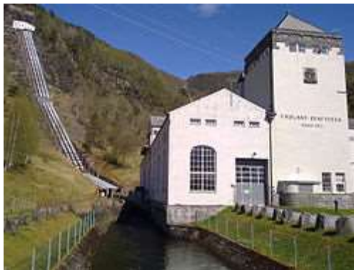
Frøland power station.
